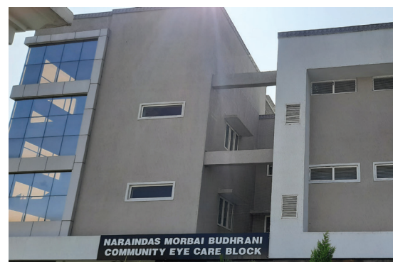
Infrastructure support for eye care facility
